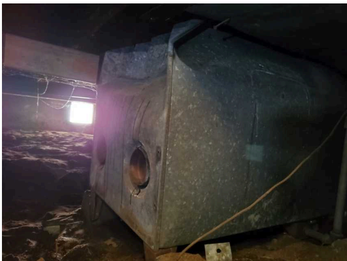
Abandoned floor furnace
