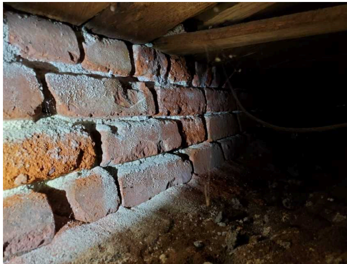
Mortar has dusted out
