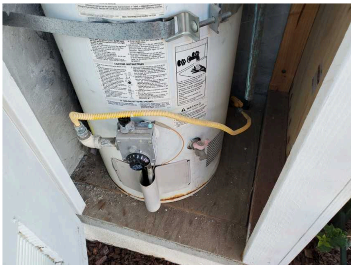
Missing sediment trap
