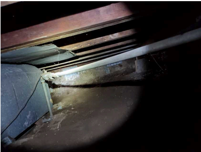
Fuel line attached to abandoned heater
