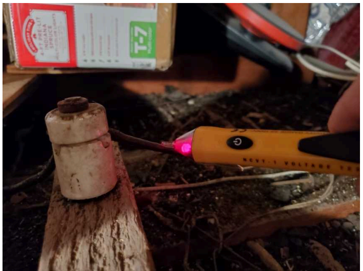
Energized K&T wiring
