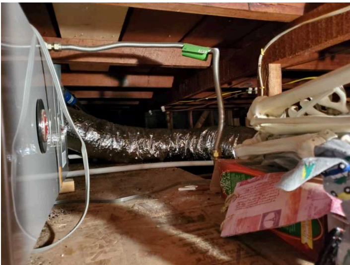
Missing sediment trap
