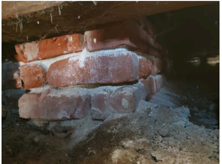
Mortar has dusted out
