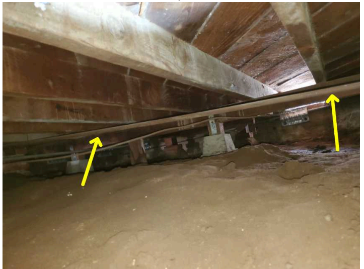
Fuel line not properly supported
