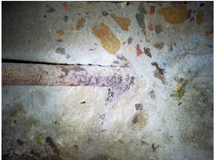
Fuel line rusted and not properly sleeved/protected
