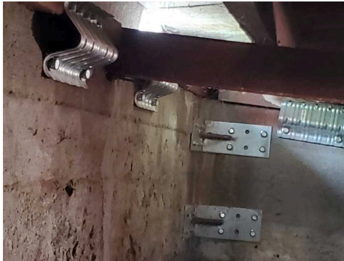
Retrofit seismic bracing and foundation wall reinforcing
