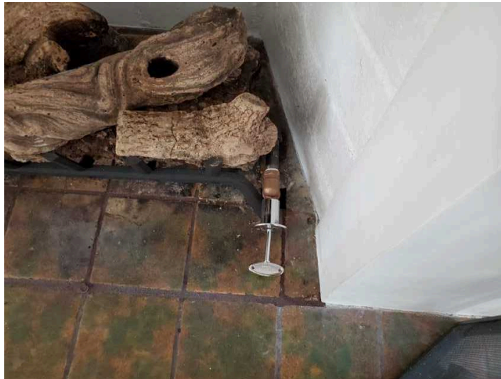
Gas valve inside firebox
