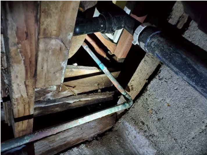
Rotted wood and missing subfloor below tub
