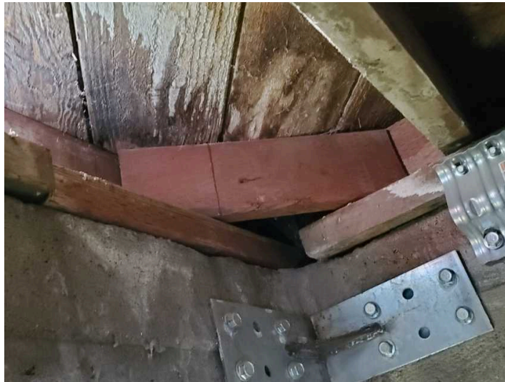
Repairs at rear right corner of house subfloor and sill plate
