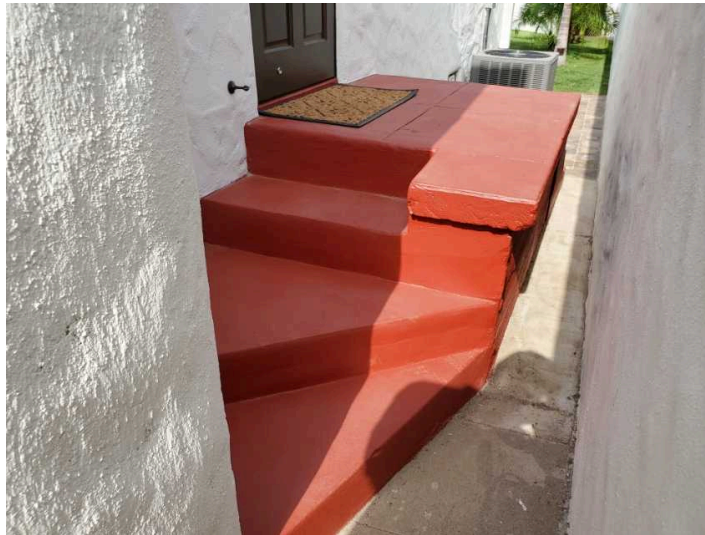
Handrail missing
