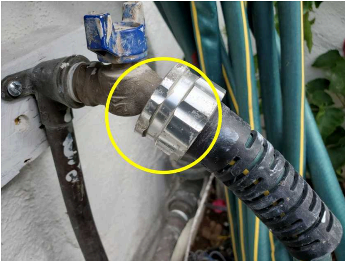
Missing anti-siphon valve
